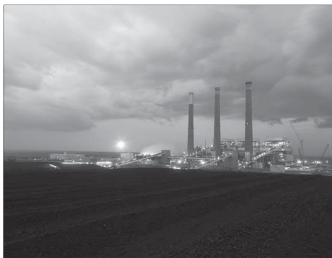
Jeffrey Energy Center near St. Marys, KS
