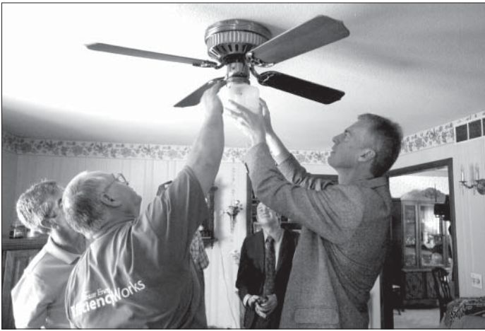
Lt. Governor Mark Parkinson helps install a compact fluorescent light bulb (CFL) at a Colwich residence during the Colwich Switch. The Colwich Switch is a partnership between Westar Energy's EfficiencyWorks division and residents in the town of Colwich. Westar provided each Colwich residence with six CFLs and will monitor the town's energy usage for one year to determine how much of a reduction in energy use occurs.
